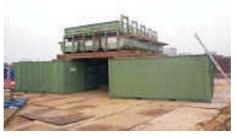
During the disposal of aircraft bombs, a protective structure is used. This structure has been tested by TNO.
